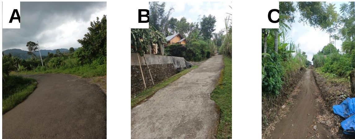
Figure 2. Road conditions by type: (a) Asphalt road, (b) Concrete road, and (c) Dirt road.
